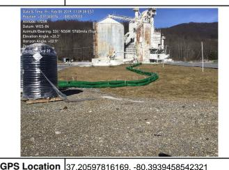
37.20597816169, -80.3939458542321 See photo for station number and GPS location. Triple stack 18 inch compost filter Description sock in place.
