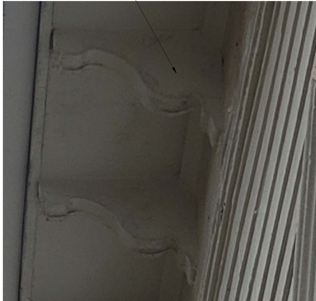
CLOSE-UP REPLACEMENT BRACKET
