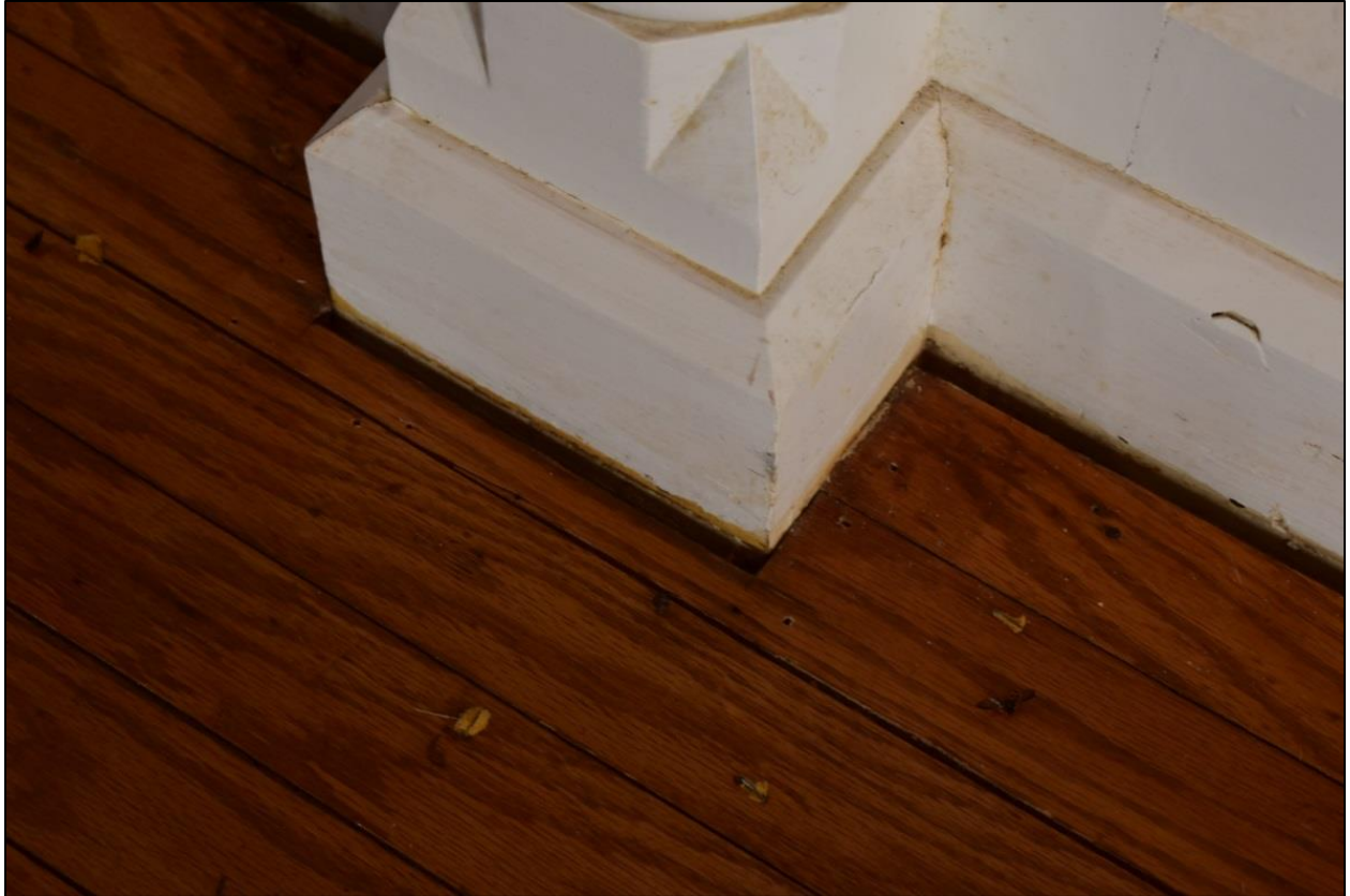
Photo 3.4.3-7. Missing quarter-round trim at bottom of main altar where carpet was removed. View Northeast.
