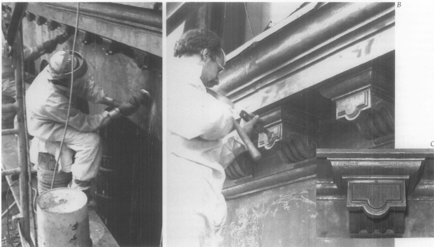
Fig. 13. Surface preparation may involve several different techniques. Where chemical paint stripping is involved, careful planning of the sequence of work and inspection by an architect or conservator to ensure strict compliance with the contract documents is important to minimize the risk of problems. After the chemical paste and paint was scraped off, the remaining paint and chemical residue were removed with a wire brush (a) and scrapers selected or cut to fit the shape of the iron surfaces (b). The surface was then wiped with solvent to create a completely clean surface prior to repainting (c). Photos: Raymond M. Pepi, Building Conservation Associates.
