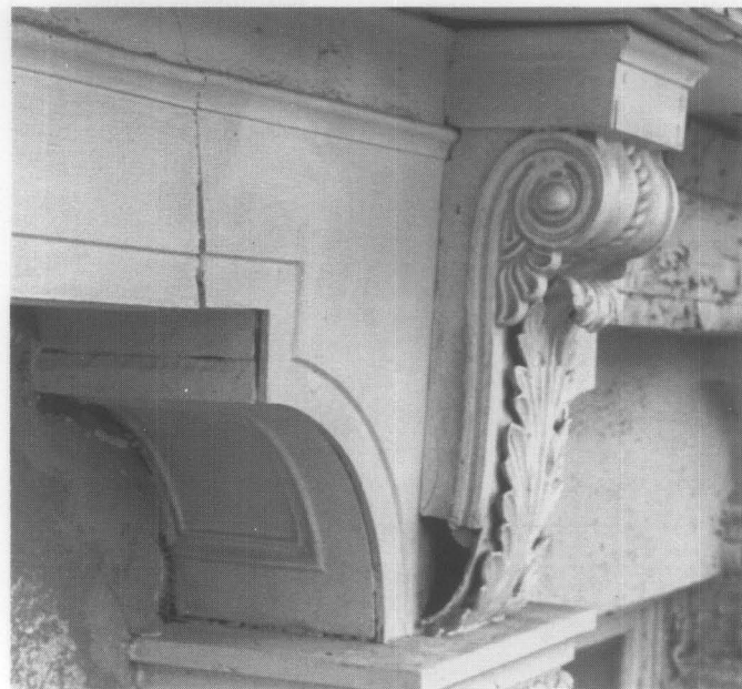
Fig. 8. Structural cracks, gaps at joints between components, and a large opening where part of the console bracket is missing are the problems evident in this cast-iron assembly. Photo: Ford, Powell & Carson.
