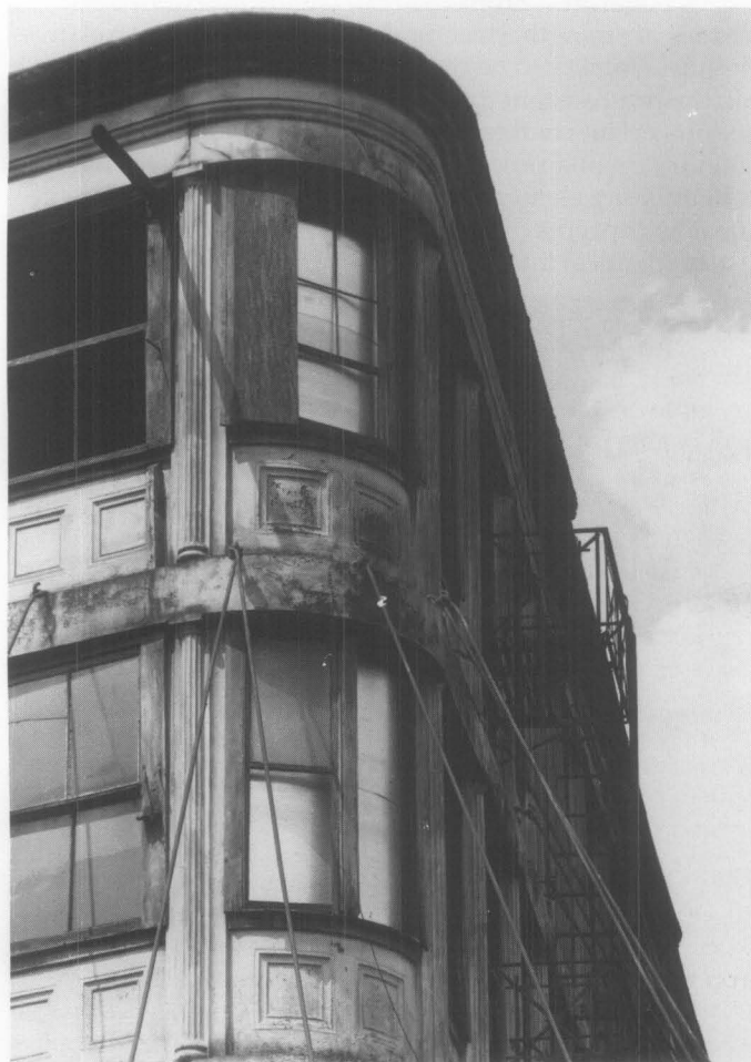
Fig. 2. The Edgar Laing Stores Block in New York City was designed by James Bogardus. It was the first building constructed with facades of self-supporting cast iron. This corner view shows the Doric-style engaged columns, panels, and spandrel beams; the loss of most of the original ornamental castings give it an austere look. As part of an urban renewal project, the facades were carefully disassembled in 1971 for later re-erection in another location—only to have its iron parts stolen for scrap. Photo: Jack E. Boucher, HABS Collection.
