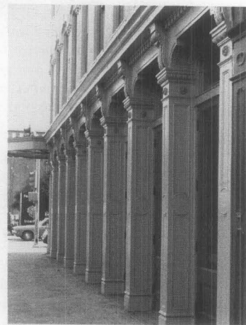
Fig. 16. Architectural cast iron is made of many small components bolted and screwed together. (a) This exploded view of a storefront illustrates the variety of elements, including brackets, fasteners, and holes for bolts. (b) The storefront was replicated in cast iron because of the extensive damage and structural failure, a detail of which is shown in Fig. 11. Drawing and photo: Historical Arts & Casting, Inc.
