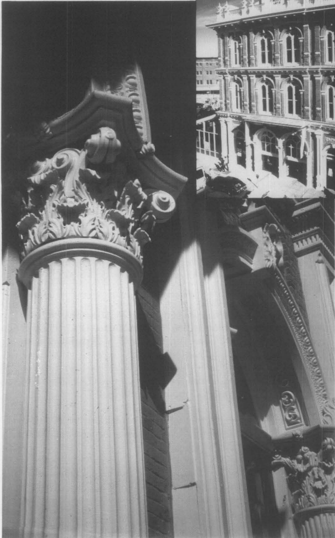
Fig. 19. (a) Fiberglass columns and aluminum capitals were installed to replicate the ornamental features on the east facade of the New Market Theater in Portland, Oregon, that had been destroyed by previous occupants. Like cast iron, crisp ornamental details can be achieved with cast aluminum. Although aluminum may be in contact with fiberglass, galvanic corrosion may result when aluminum is in direct contact with cast iron. Photo: William J. Hawkins, III. (b) The west facade of the theatre retains its original cast iron features. Photo: George McMath.
