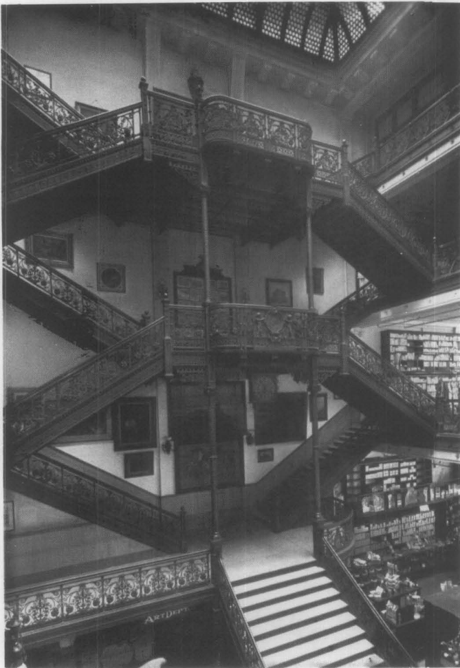
Fig. 4. The 1904 grand stairway of the former Frear's department store in Troy, N.Y. was constructed of cast iron, as was the frame of the skylight above. Some ornamental wrought iron was also employed. This use of iron was typical in major commercial buildings constructed throughout the United States. Courtesy: Rensselaer County Historical Society.
