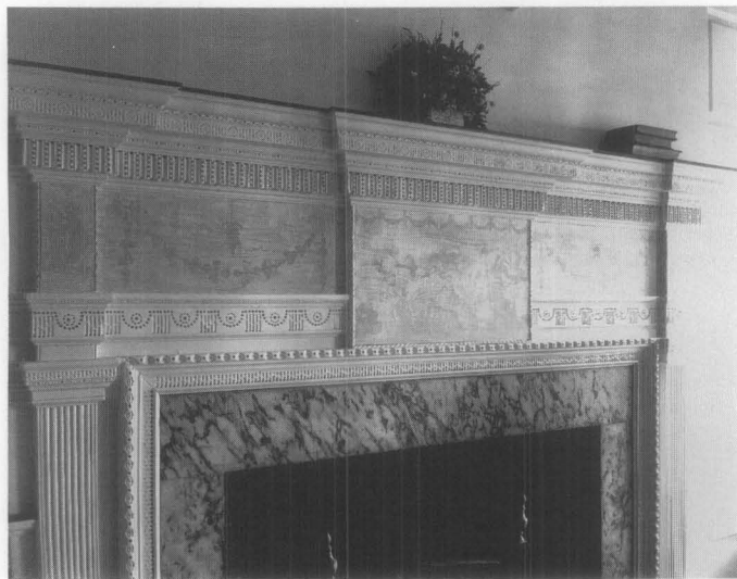
Figure 29. The ghost marks of compo past—floral swags or festoons—are in clear evidence on a mantelpiece in the back bedroom of the George Read II House, New Castle, Delaware. This physical evidence will be used to assure their accurate re-creation in a restoration project. Photo: Courtesy, Gold Leaf Studios, Inc.
