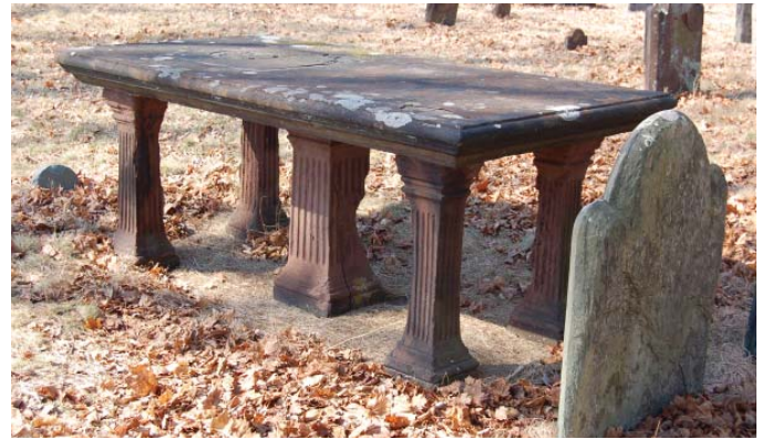
Figure 4. This sandstone table tomb, located in Cedar Grove Cemetery, New London, CT, is an engineered grave marker structure consisting of a horizontal stone tablet supported by four vertical table "legs" with and a central column,. Photo: Jason Church.
