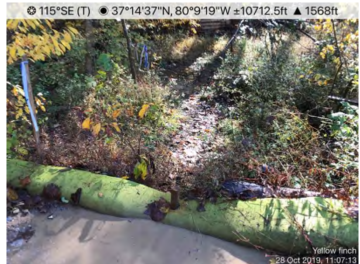
Fig. 4: MVP-MN-278.01 – Yellow Finch Lane. CFS installed correctly and functioning properly at the time of inspection.
