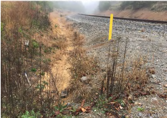
Fig. 7: STA 12197+40 – Looking NE towards RVRA spur line from ROW. Erosion along channel and banks of rail line evident.
