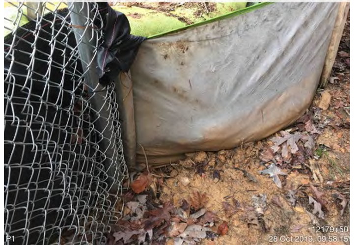
Fig. 8: STA 12179+50 – P1 undermined. Maintenance needed
