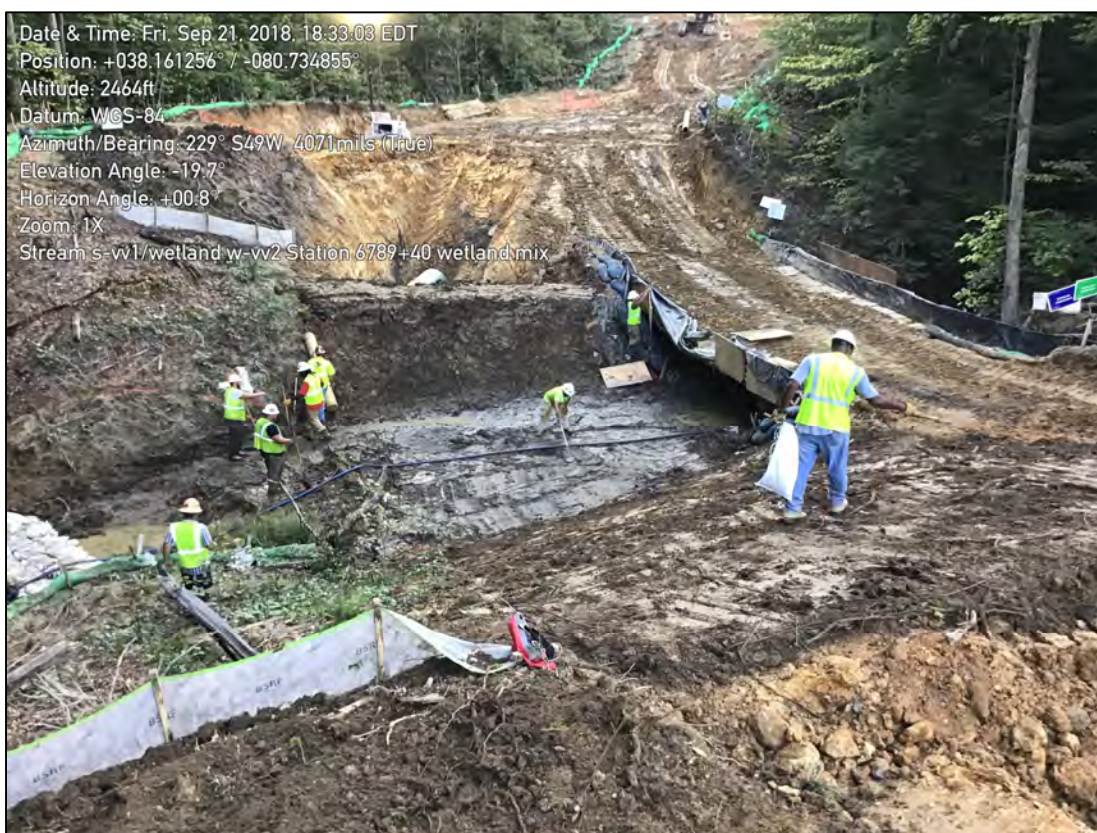
Photo illustrates the construction conditions of stream S-VV1 and wetland w-VV2. Note that the water has been completely diverted during construction.
