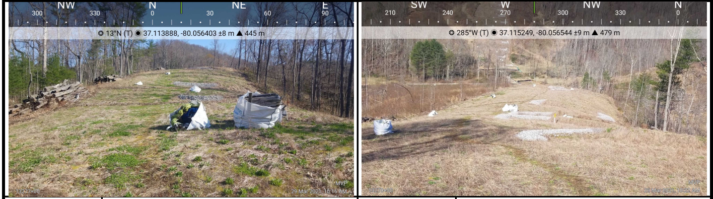
GPS Location See photo coordinates. GPS Location See photo coordinates. Field Station# 13277+00 Field Station# 13270+00 Pic 5 Desc. ROW stable with vegetative cover across LOD. Pic 6 Desc. ROW stable with vegetative cover across LOD.
