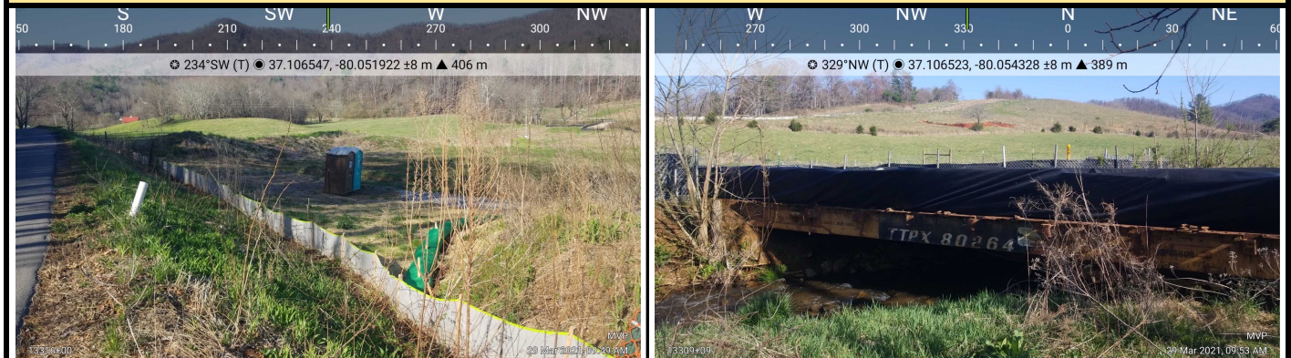
GPS Location See photo coordinates. GPS Location See photo coordinates. Field Station# 13316+00 Field Station# 13309+00 Pic 1 Desc. CIS of Wades Gap, perimeter controls in acceptable condition along road crossing. Pic 2 Desc. S-GH7, upstream, bridge in good condition, no changes noted at stream crossing.
