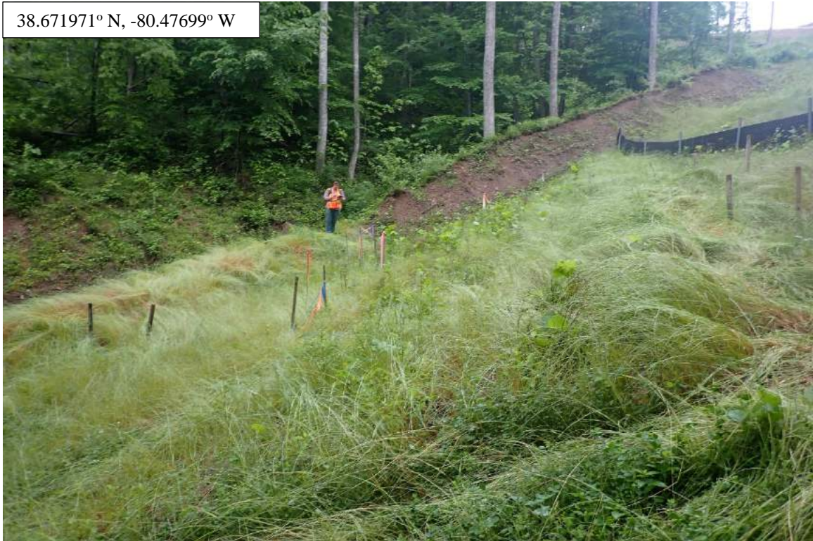
Photo Type: UG View of Location in Shapefile Location, Orientation, Photographer Initials: Upgradient View of Location in Shapefile, ABK/BB
