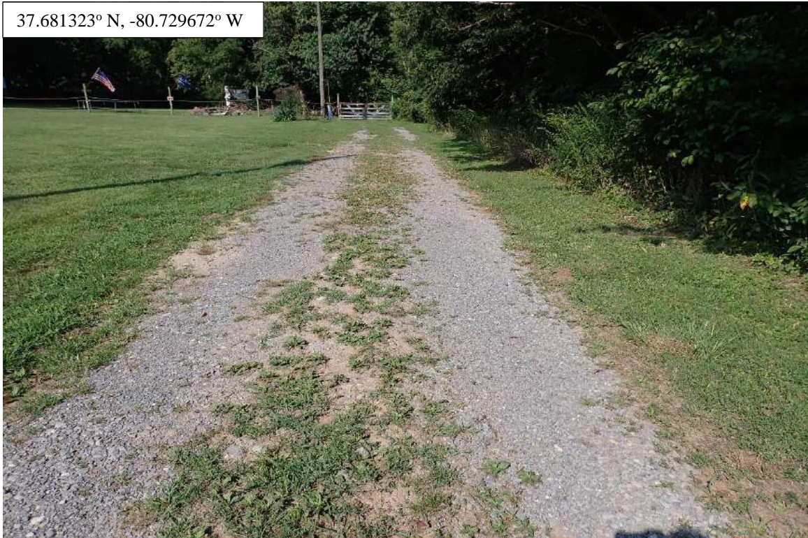
Photo Type: View Up the AR Location, Orientation, Photographer Initials: View Up the Access Road, AK/RA/TA
