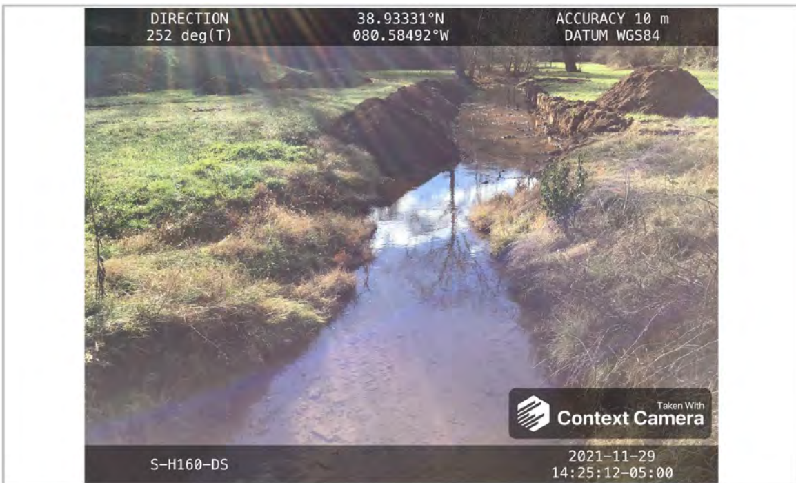
Photo Type: Downstream View Location: 38.93331, -80.58492 Photo Orientation: W (252 degrees) Stream Type: Plane bed Notes: Earth disturbance not associated with the MVP Project
