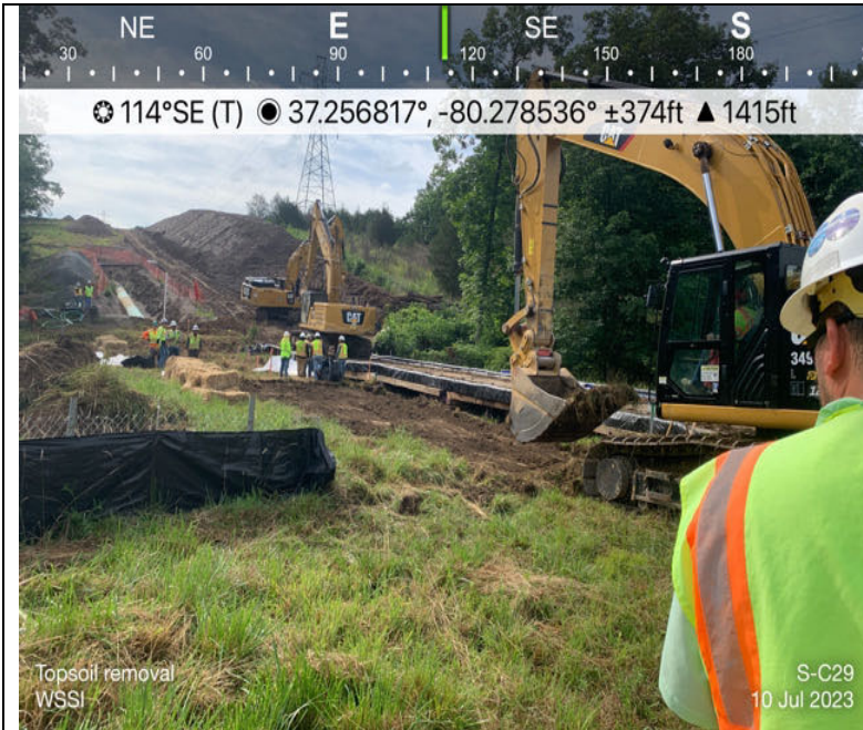
Photo Description: Topsoil removal.
