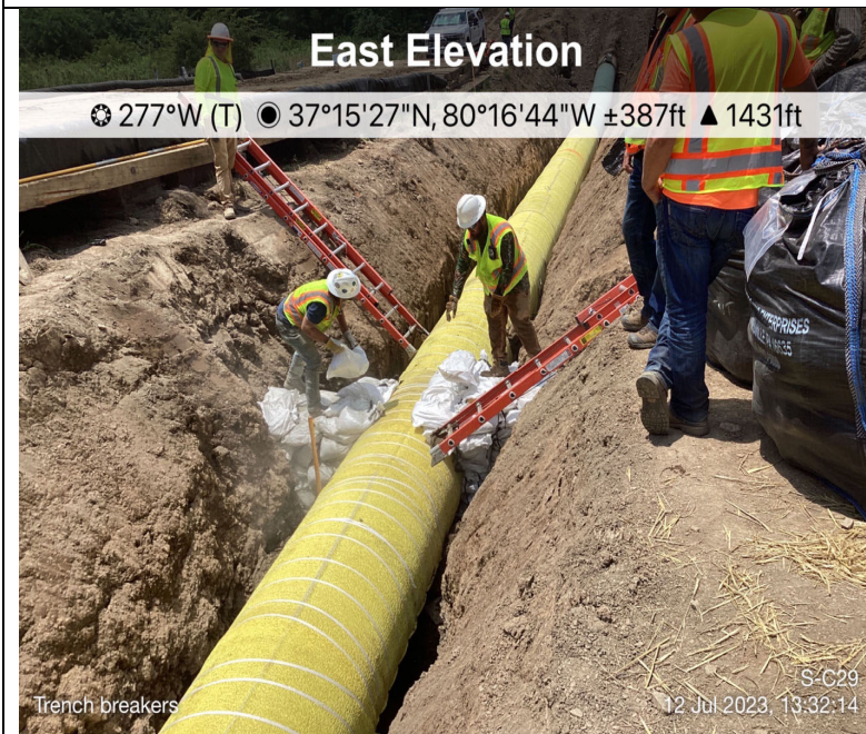
Photo Description: Trench breakers being installed.
