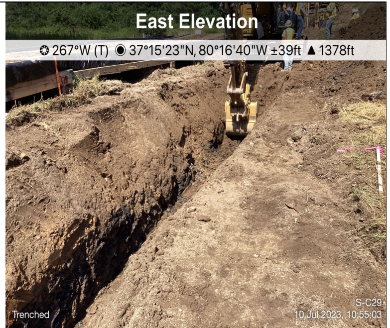
Photo Description: Trenching.
