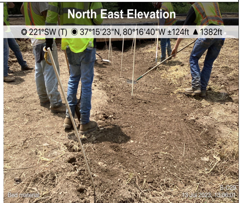
Photo Description: Stream material returned to the stream bed and fine grading.
