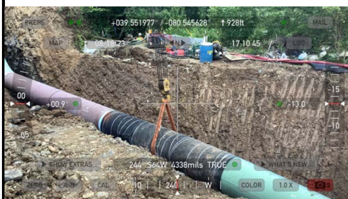
GPS Location see photo Description This photo shows the pipe installed in the water body crossing
