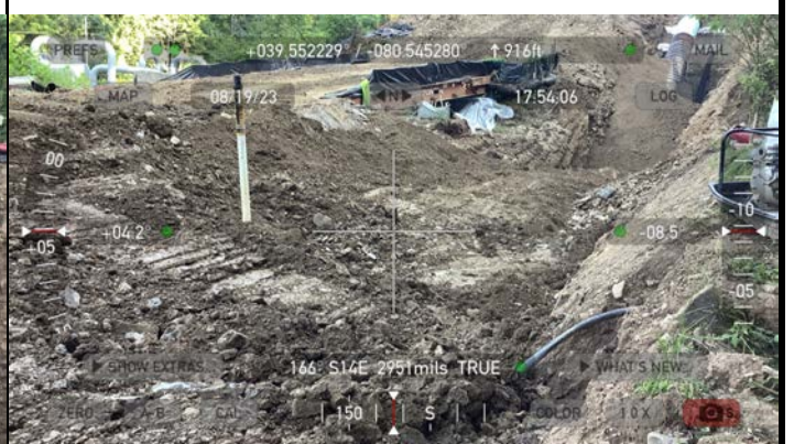
GPS Location see photo Description This photo shows the backfilled subsoil in the water body crossing prior to replacement of substrate
