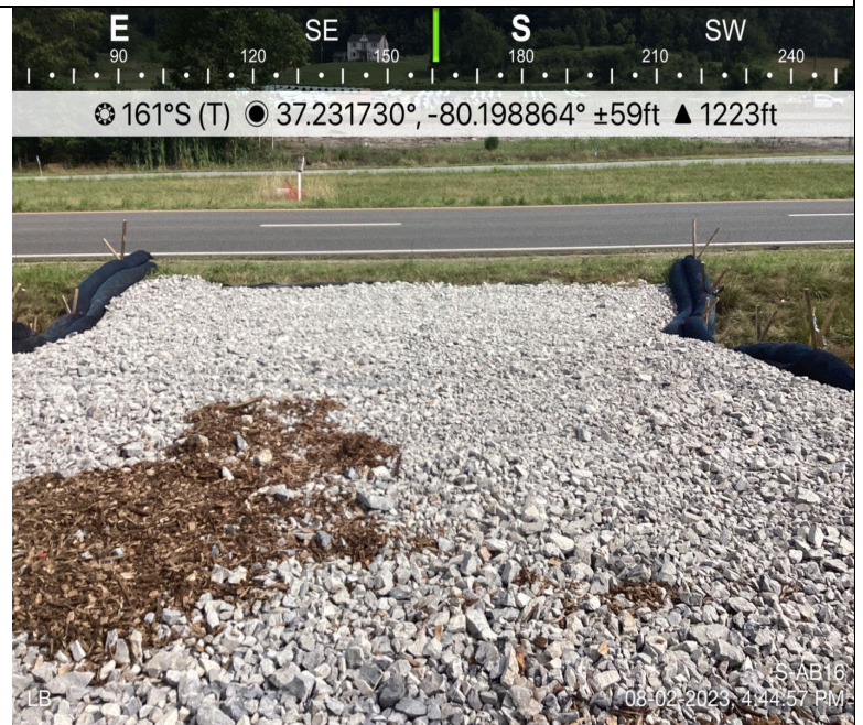
Photo Description: Left bank view during post-construction assessment.
