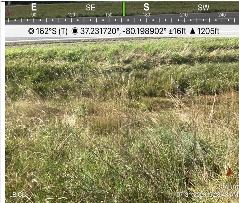
Photo Description: Left bank view during pre-construction assessment
