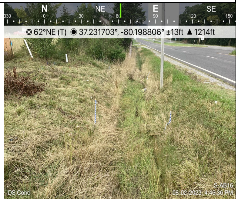
Photo Description: Downstream view of unpermitted area during post-construction assessment.
