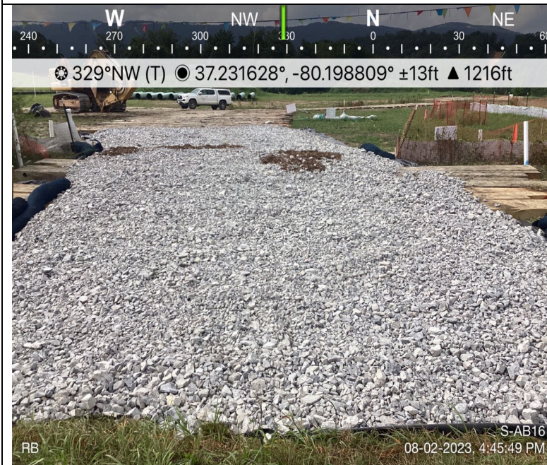
Photo Description: Right bank view during post-construction assessment
