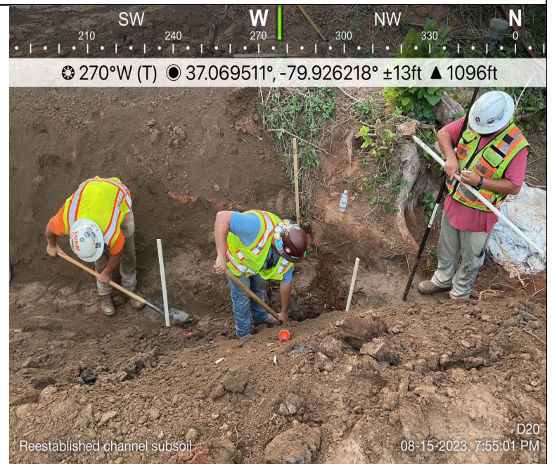
Photo Description: Fine grading of stream channel.
