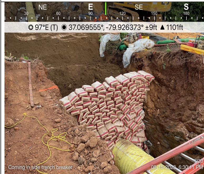
Photo Description: Bentonite trench breaker on coming in side of S-D20.
