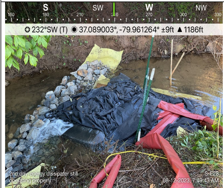
Photo Description: Downstream energy dissipator.
