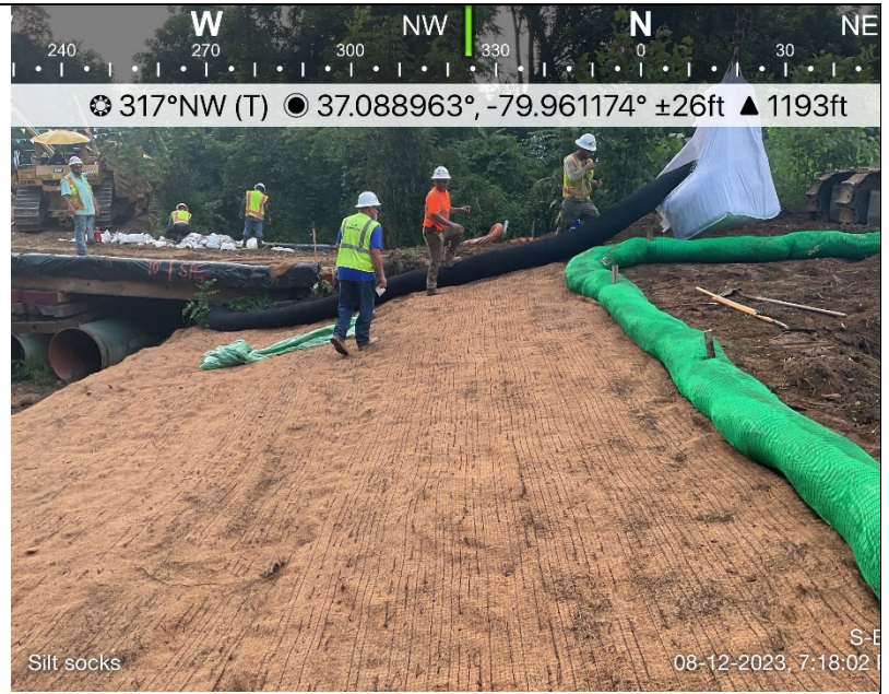
Photo Description: Erosion control matting on banks.
