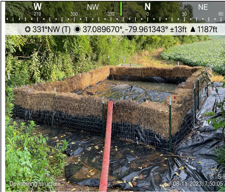
Photo Description: Dewatering structure.
