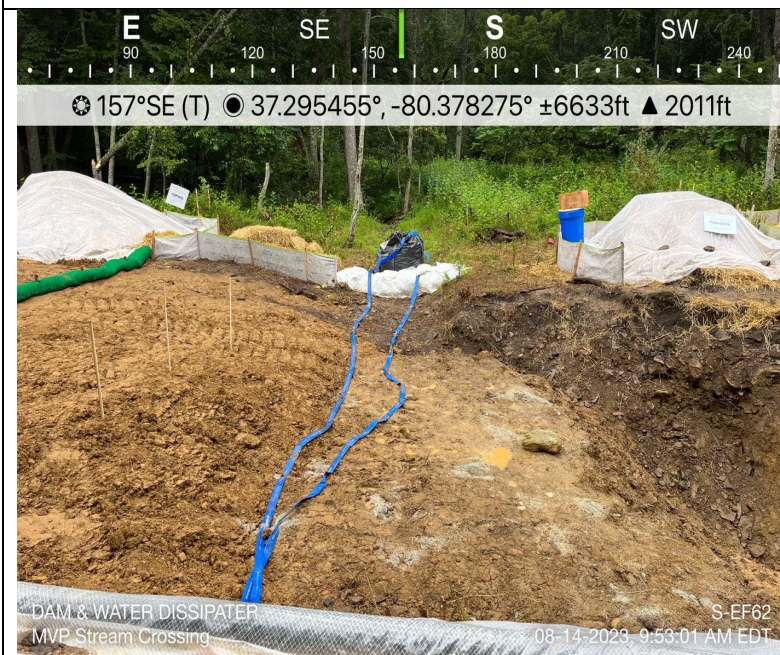
Photo Description: Dam Energy Dissipator and topsoil stockpiles.
