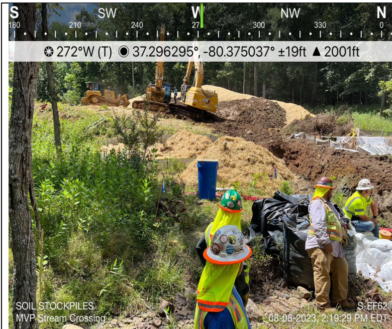
Photo Description: Soil Stockpiles
