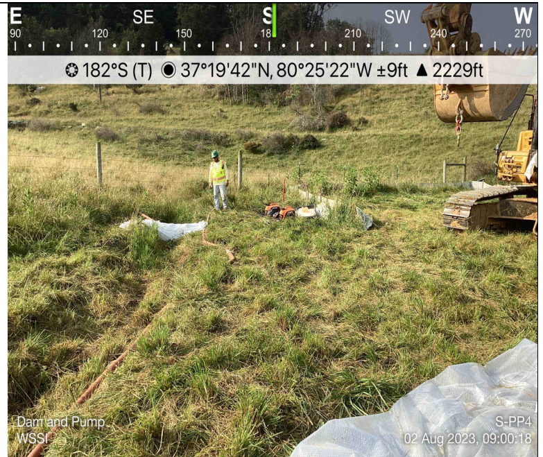
Photo Description: Dam and pumps in place and functioning.
