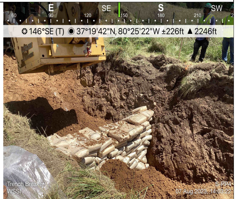
Photo Description: Trench breakers installed and backfilling underway.
