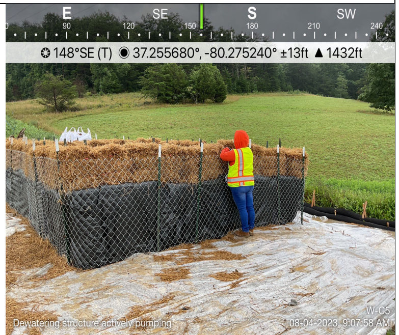
Photo Description: Dewatering structure actively functioning
