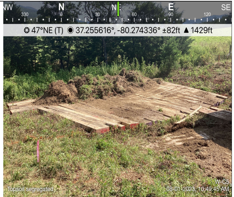
Photo Description: Topsoil was segregated and placed on timber mats
