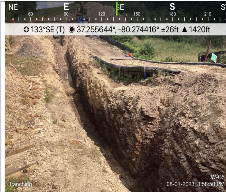
Photo Description: Trenching complete with keys cut for trench breaker
