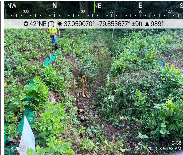
Photo Description: Upstream view of resource prior to construction.
