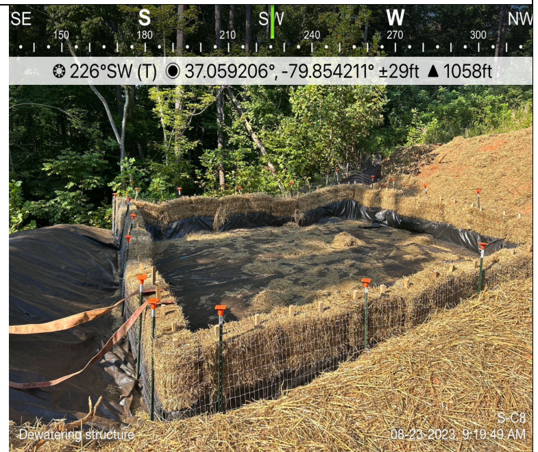
Photo Description: Dewatering operation set up for use, as needed.
