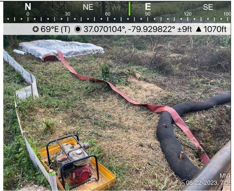
Photo Description: Trench dewatering area
