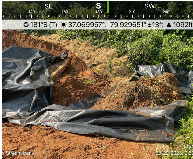
Photo Description: Topsoil Stockpile
