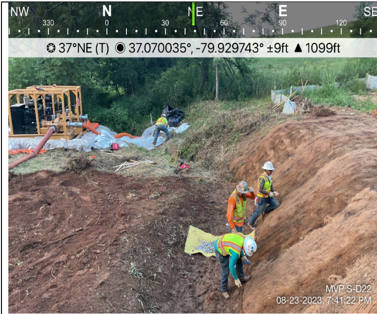
Photo Description: Bank stabilization and pump around
