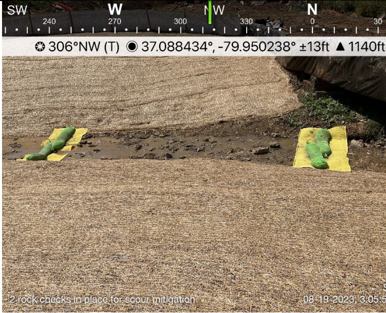
Photo Description: Temporary check dams to slow initial flows returning to stream
