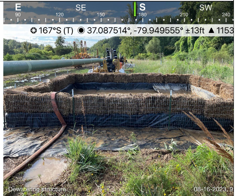
Photo Description: Trench dewatering area.
