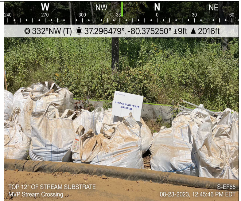
Photo Description: Stream substrate stockpile
