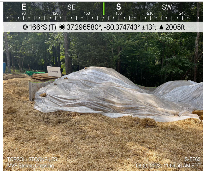
Photo Description: Topsoil stockpiles
