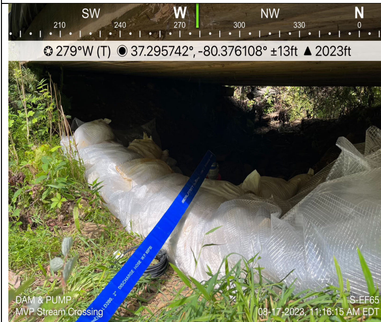
Photo Description: Dam & pump
