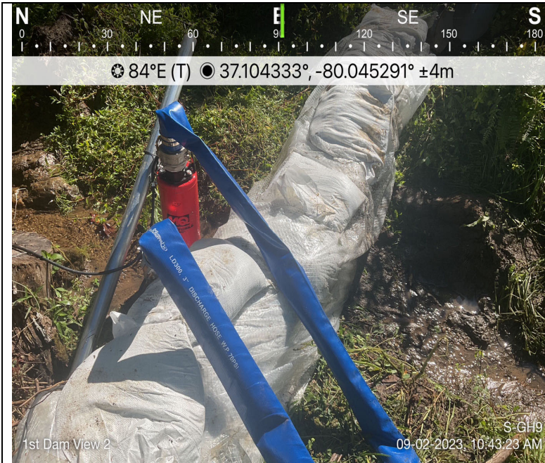
Photo Description: Upstream dam placed in stream.
