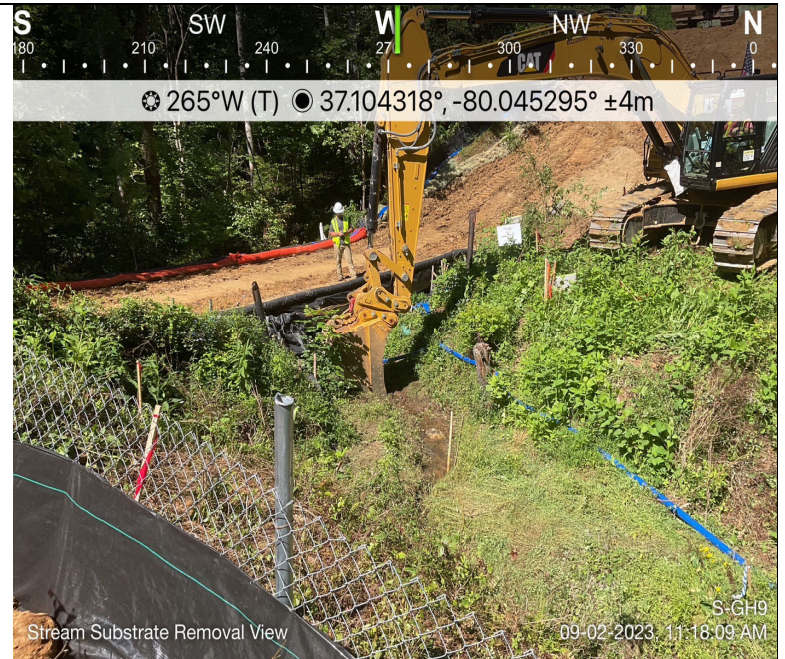
Photo Description: Stream substrate removal and segregated away from trench materials.
