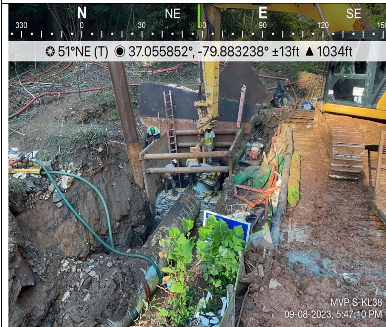
Photo Description: Trench breakers being installed.
