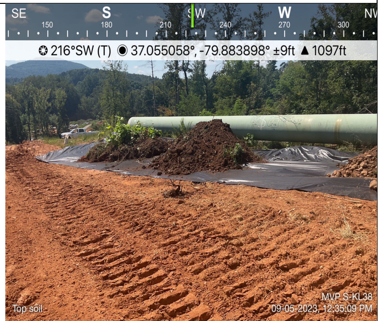
Photo Description: Top soil stockpiled separately.
