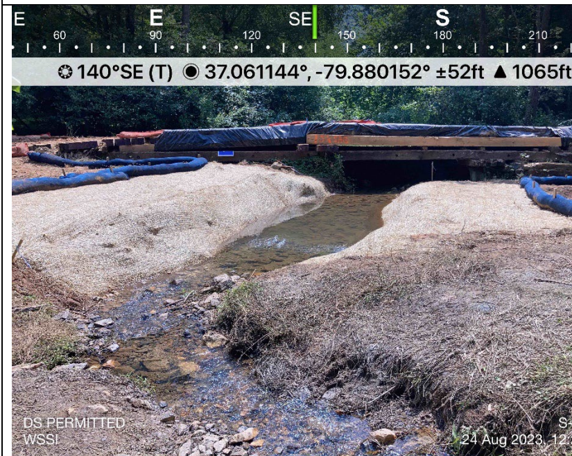
Photo Description: Downstream view of permitted impact area during post-construction assessment.
