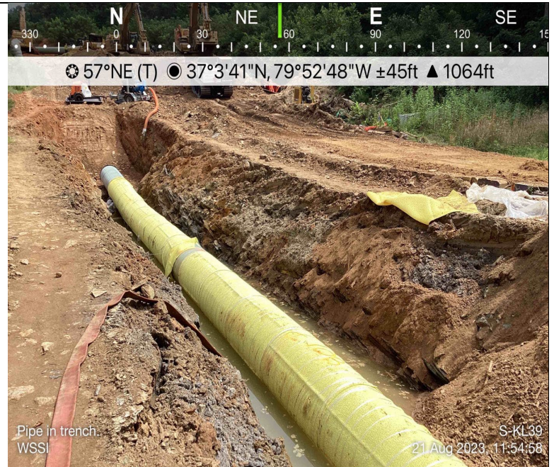
Photo Description: Pipe in trench.
