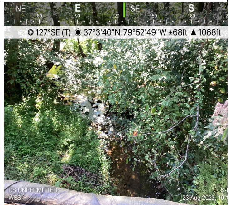
Photo Description: Downstream view of unpermitted area during post-construction assessment.
