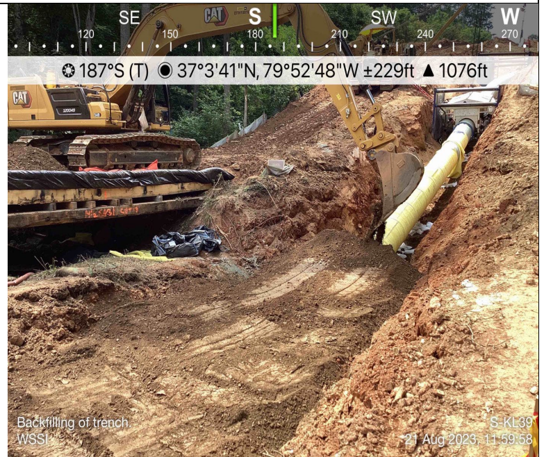
Photo Description: Backfilling of trench.
