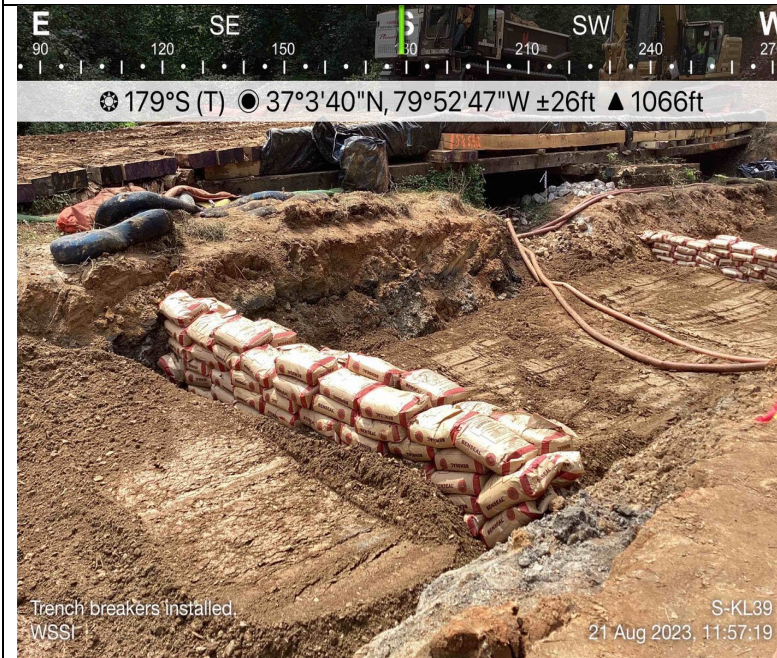
Photo Description: Trench breakers installed.
