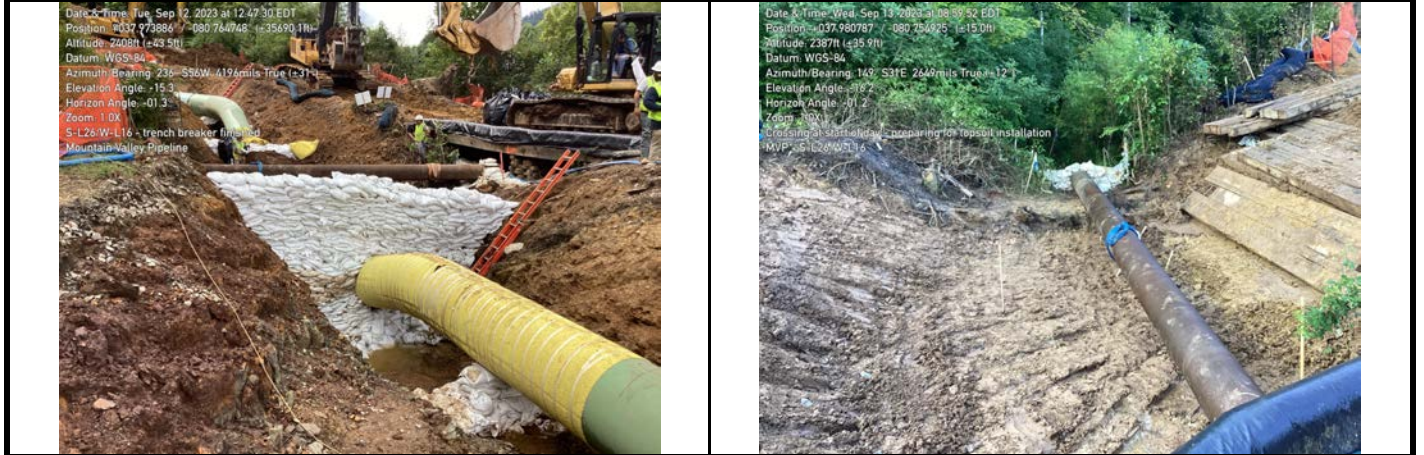
GPS Location See Photo GPS Location See Photo Description Photo 5: Trench breakers at aquatic resources. Description Photo 6: Contouring the stream channel.
