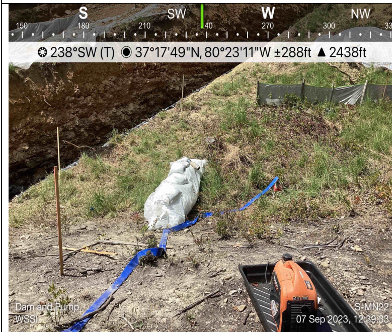
Photo Description: Dam and pump in dry stream.
