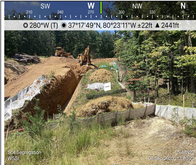
Photo Description: Soil segregation in buffer areas.
