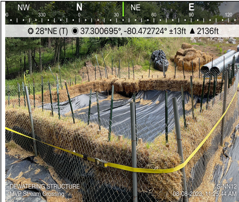
Photo Description: Dewatering structure.
