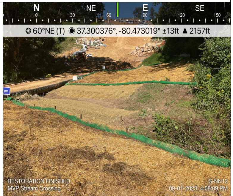
Photo Description: Stream restoration finished.
