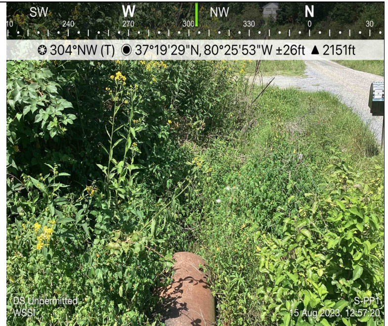
Photo Description: Downstream view of unpermitted area during pre-construction assessment.
