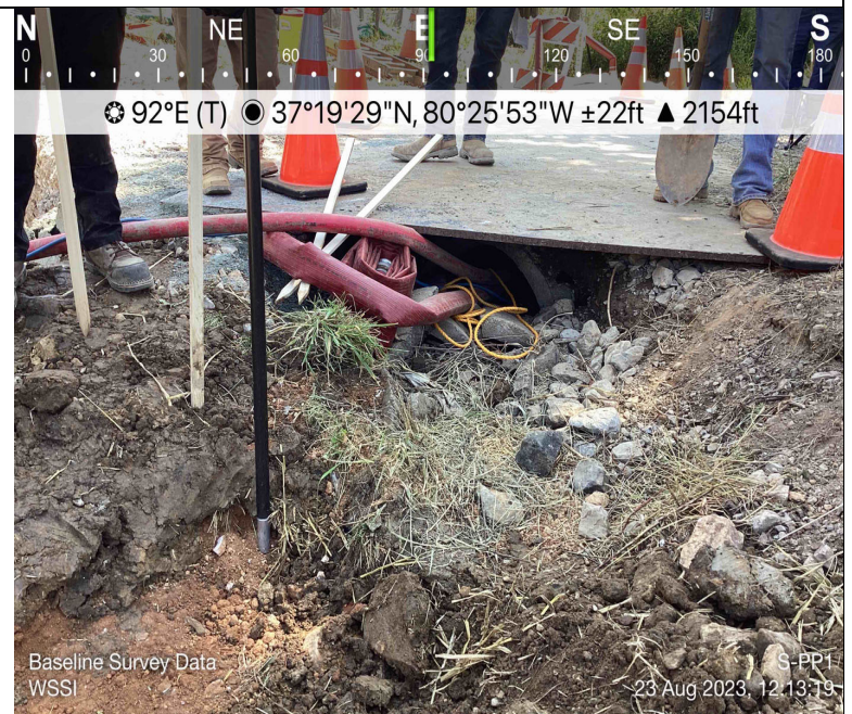
Photo Description: Baseline data survey did not match up to current field conditions. Therefore, a modification was made to only one point, the toe of bank in cross section A. All other data points held constant.
