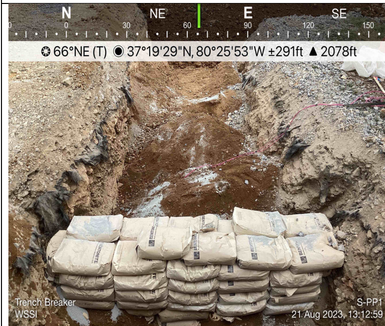
Photo Description: Trench Breakers installed appropriately.
