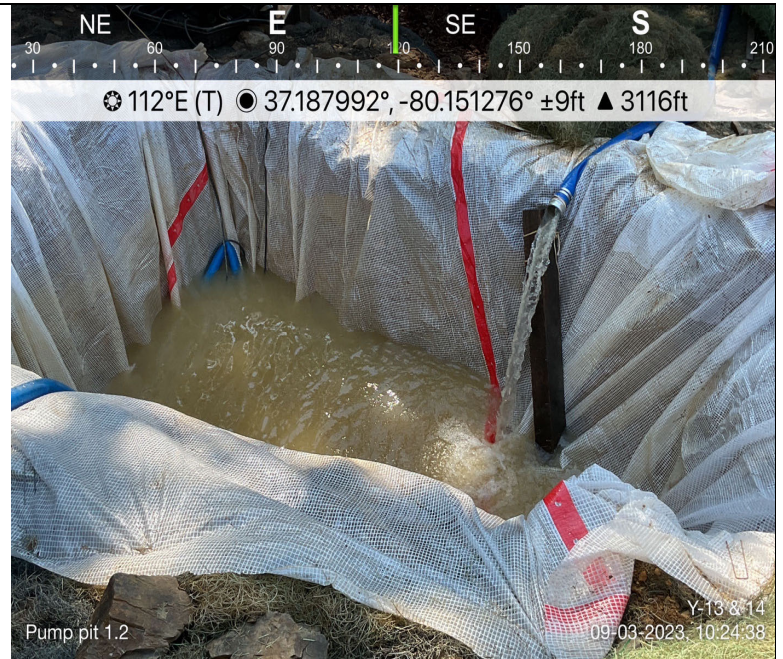
Photo Description: Dewatering pit
