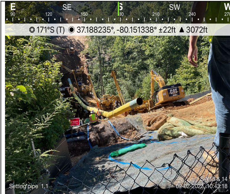
Photo Description: Setting Pipe
