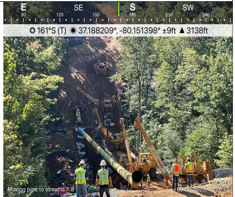
Photo Description: Moving pipe to crossing.
