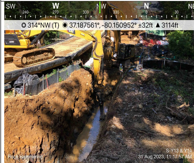
Photo Description: Trench excavation and rock hammer.
