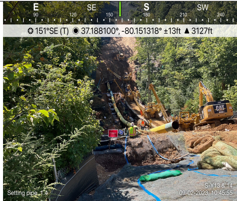
Photo Description: Pipe being set into trench.
