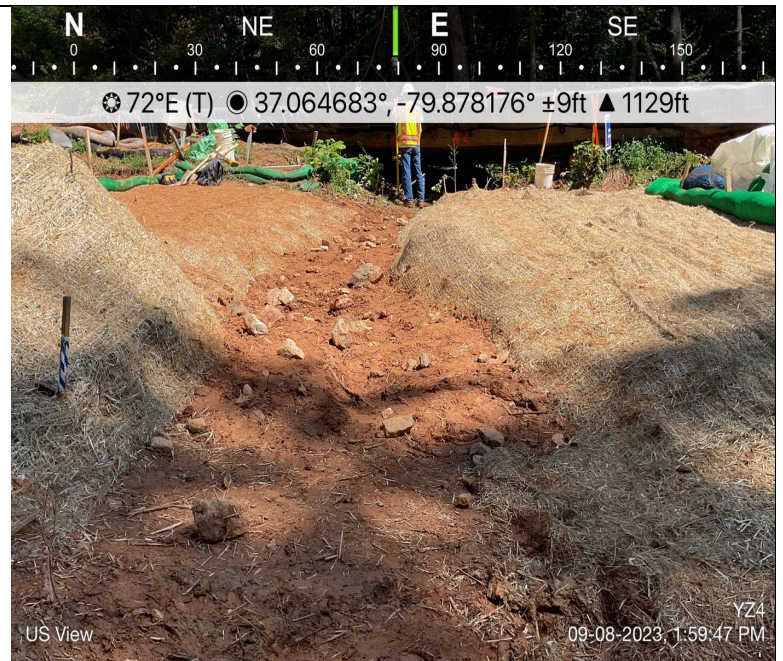
Photo Description: Upstream view of resource during restoration activities.
