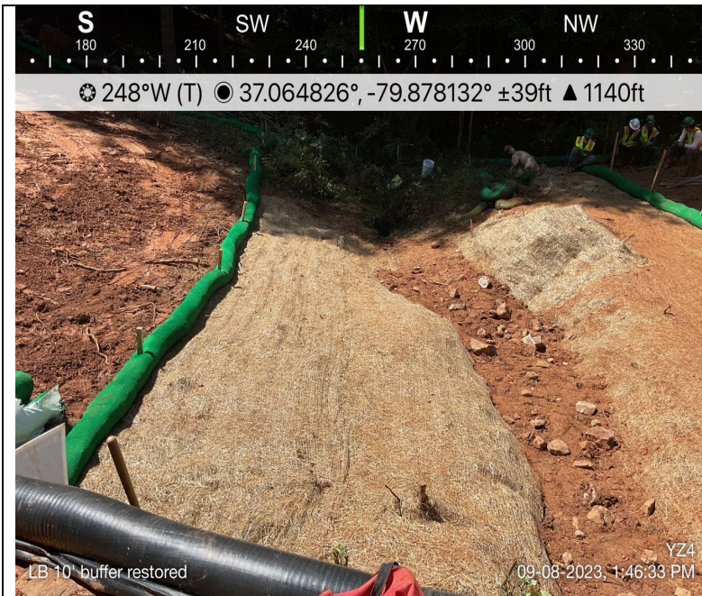
Photo Description: Restoration of left bank within FERC 10' buffer.
