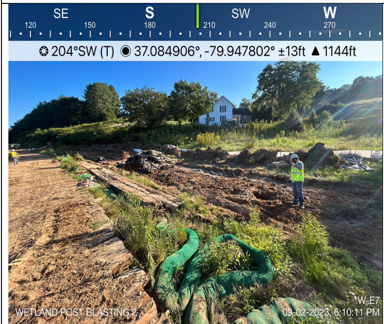
Photo Description: Wetland impact area post-blasting.
