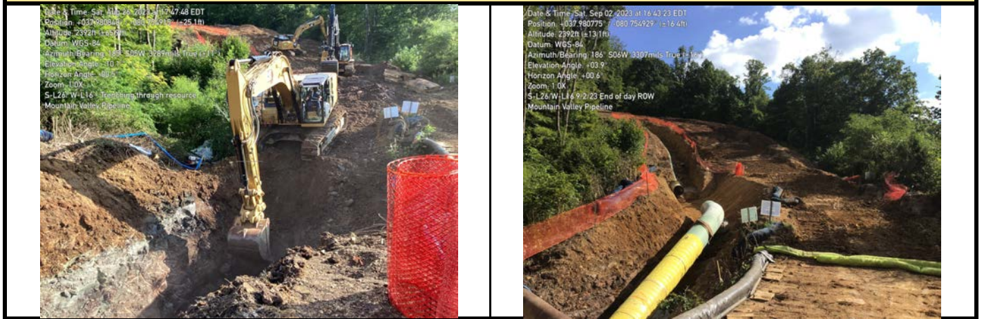
GPS Location See Photo GPS Location See Photo Description Photo 3: Trenching through aquatic resources. Description Photo 4: Pipe lowered into aquatic resources.
