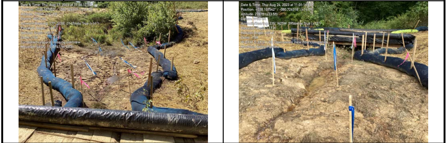
GPS Location See Photo GPS Location See Photo Description Photo 5: Surveyed and restored stream. Description Photo 6: Sinking stream (8/24/2023)
