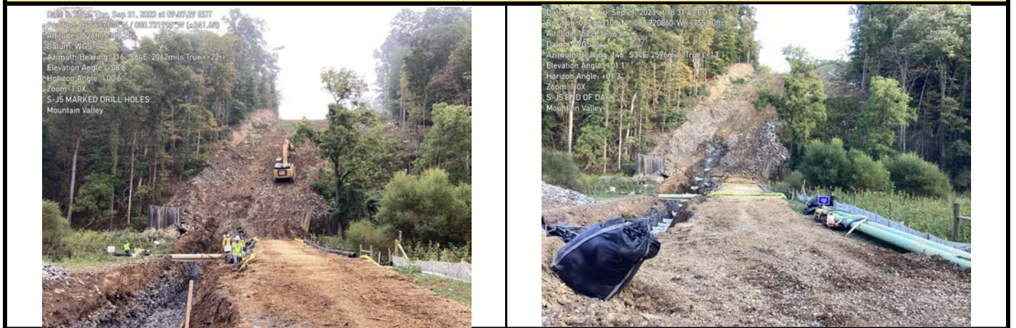
GPS Location See Photo GPS Location See Photo Description Photo 3: Trench through aquatic resource. Description Photo 4: Bedding placed in trench in aquatic resource.
