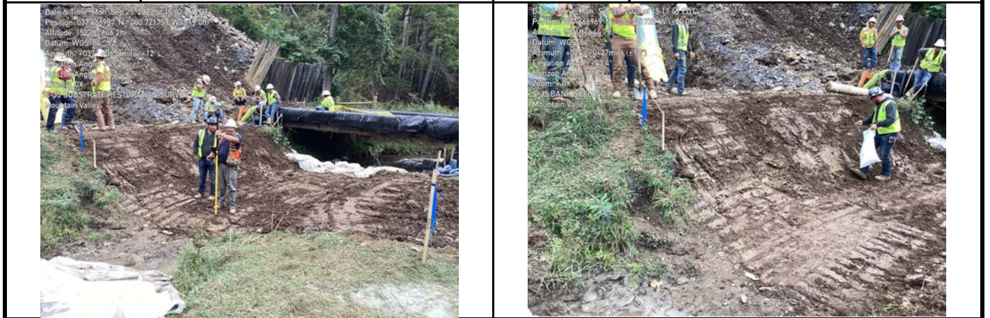
GPS Location See Photo GPS Location See Photo Description Photo 7: Substrate restoration and survey. Description Photo 8: Seeding of banks.
