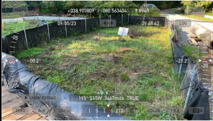
GPS Location See photo Description View of permitted resource impact area during pre-construction assessment.
