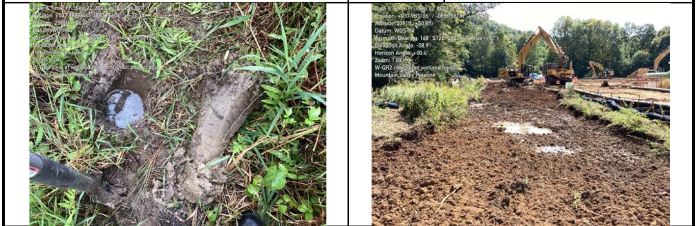
GPS Location See Photo GPS Location See Photo Description Photo 1: Soil test pit with recharge and saturated soils. Description Photo 2: Wetland topsoil removed at first resource crossing.
