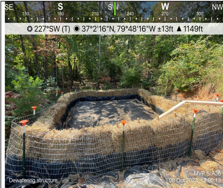
Photo Description: Dewatering structure
