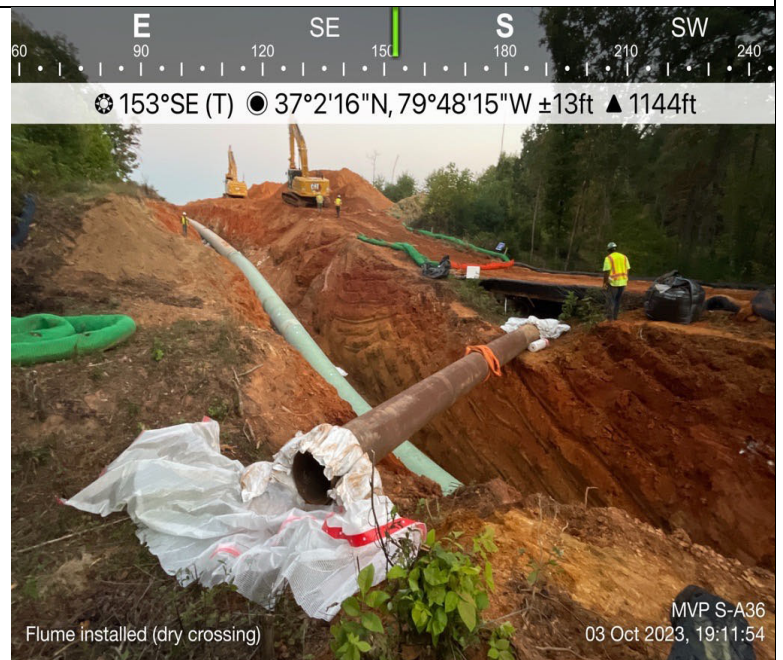
Photo Description: Flume installed
