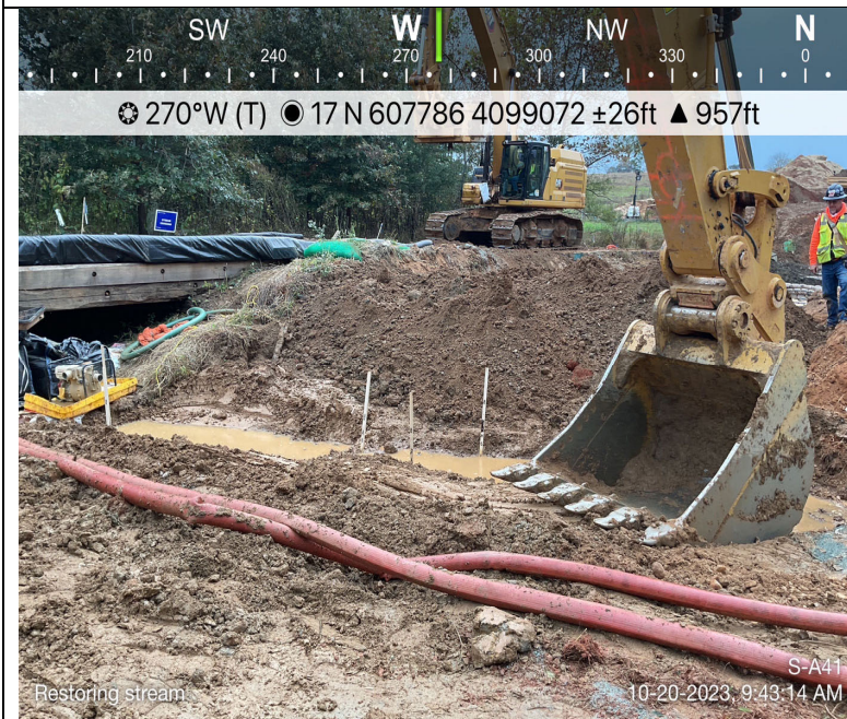
Photo Description: Restoration of the stream banks.
