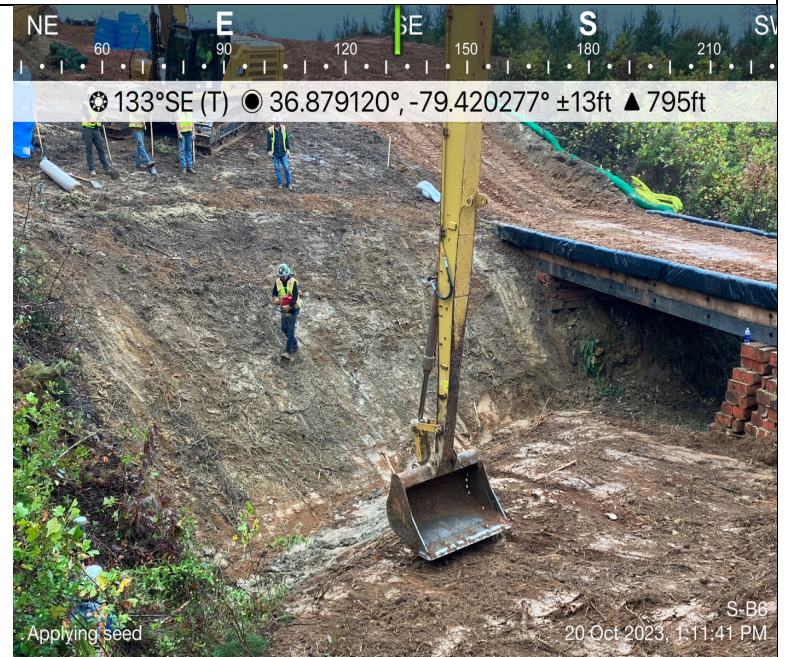
Photo Description: Restoration activities along the stream bank.
