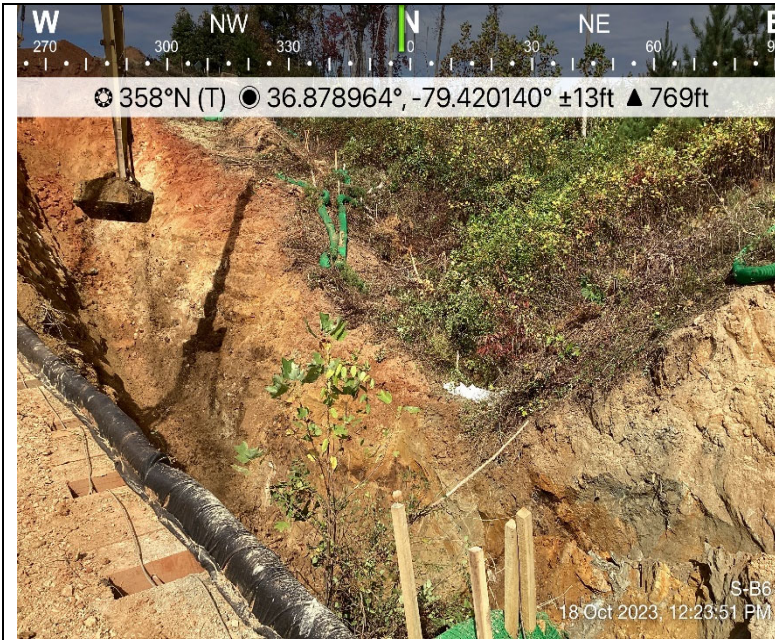
Photo Description: Excavating the trench.
