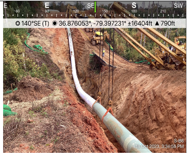
Photo Description: Pipe being lowered into the trench.
