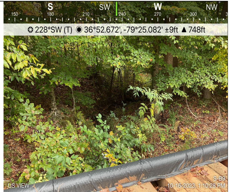
Photo Description: Conditions of the downstream area outside the ROW during pre-construction assessment.
