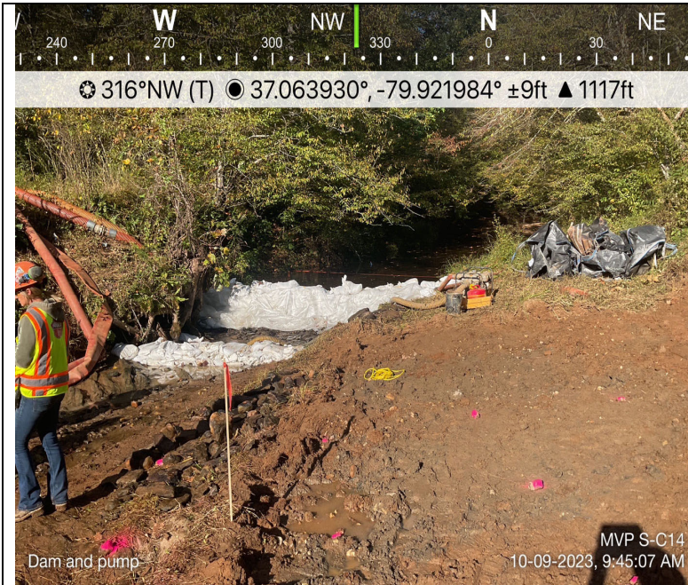
Photo Description: Dam and pump setup
