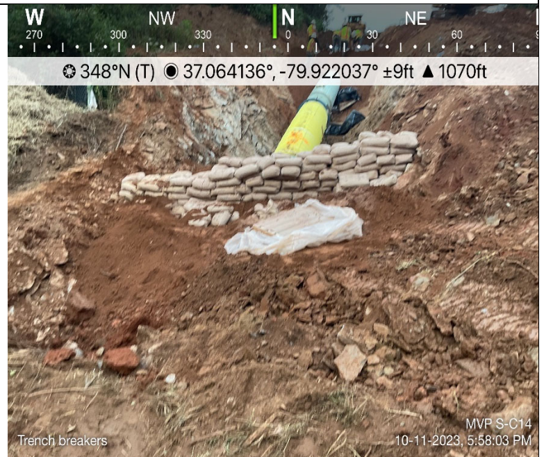
Photo Description: Trenchbreaker installed.
