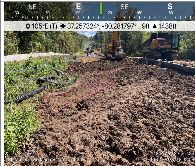
Photo Description: Survey staked stream for restoration.
