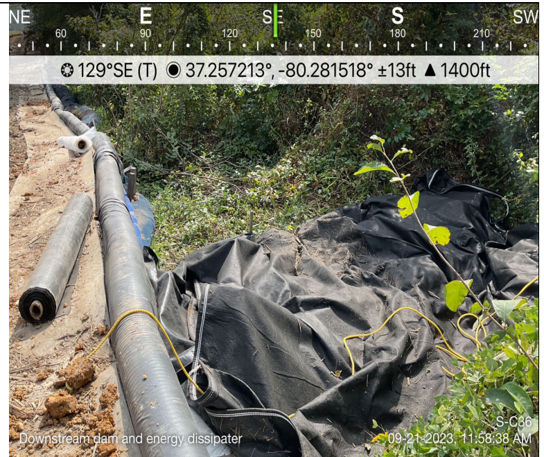
Photo Description: Downstream dam and energy dissipater.
