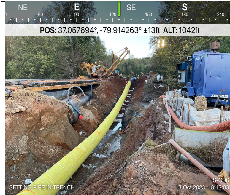
Photo Description: Lowering the pipe in the trench.
