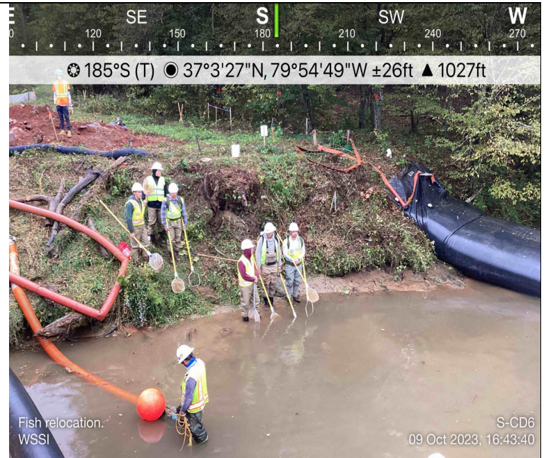
Photo Description: Fish relocation in progress.
