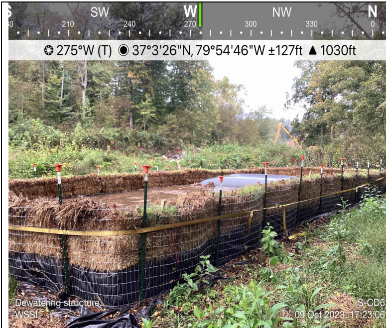
Photo Description: Overview of the dewatering operations.
