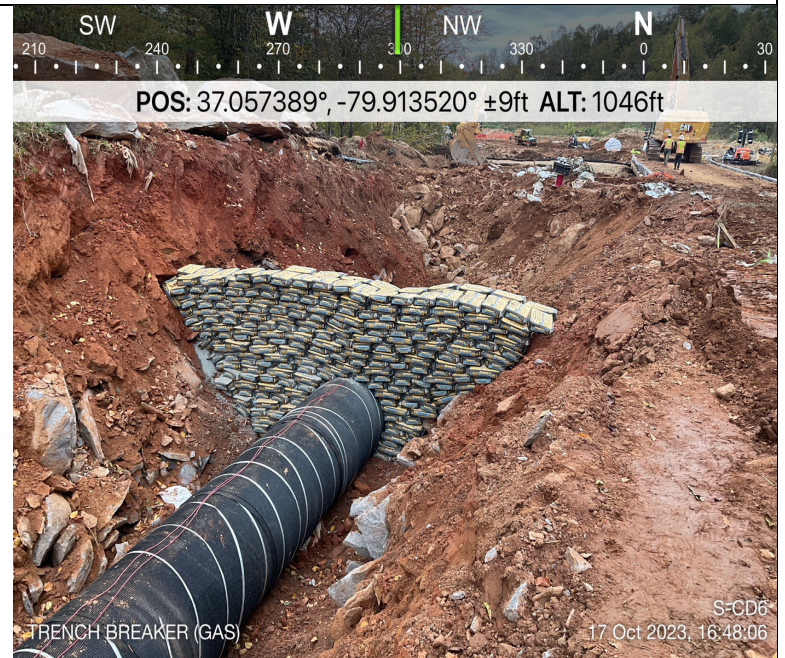
Photo Description: Trench breaker installed.
