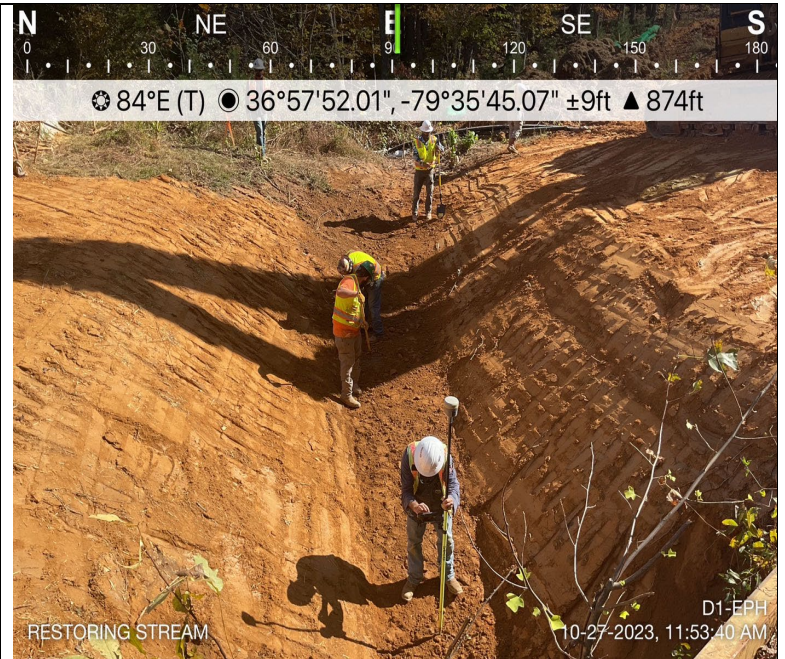
Photo Description: Surveying the stream for site restoration.
