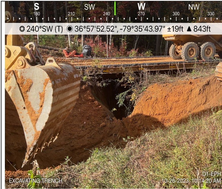
Photo Description: Excavation of the trench.
