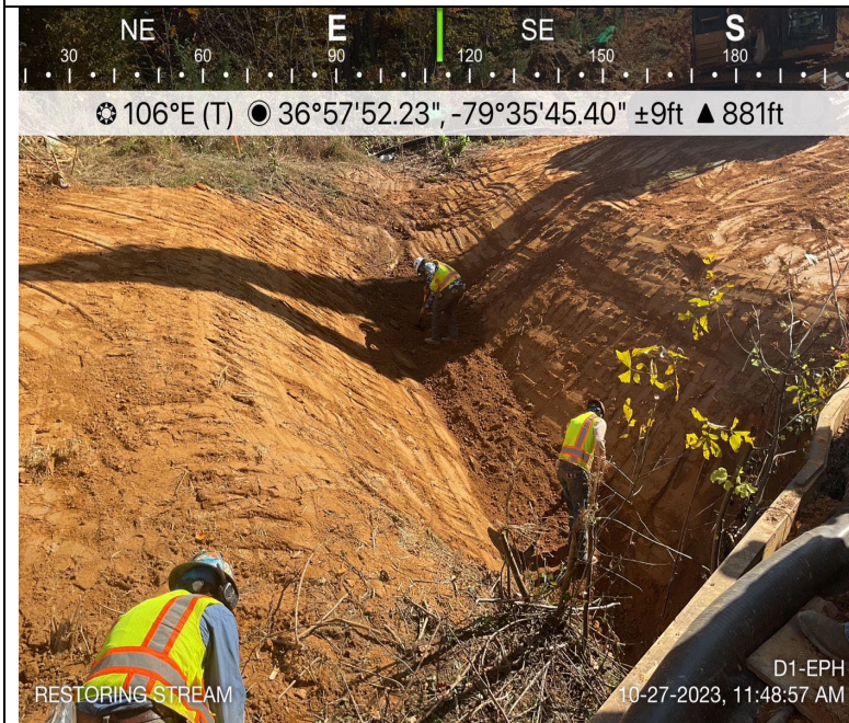
Photo Description: Restoration of the stream bed and banks.
