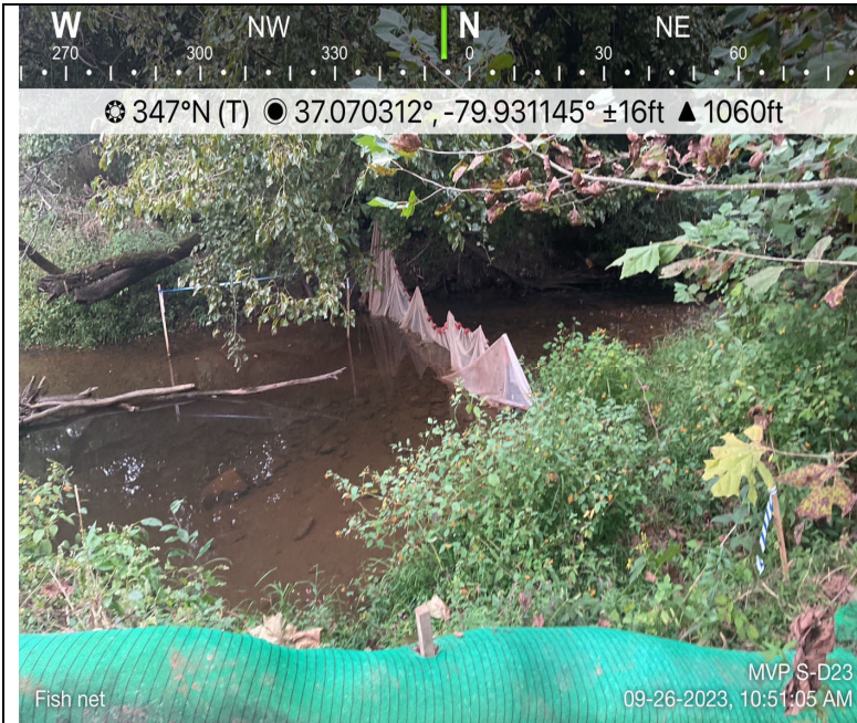
Photo Description: Fish net left in place throughout crossing to prevent fish from migrating back into impact area.
