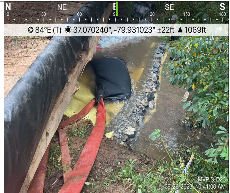
Photo Description: Pump around energy dissipator rock check.
