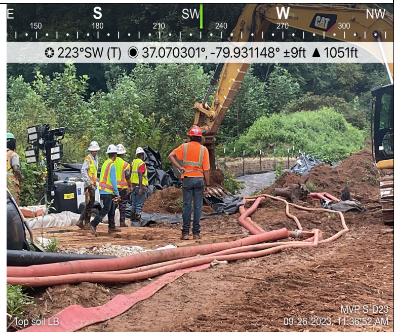
Photo Description: Left bank topsoil stockpiled separately from subsoil
