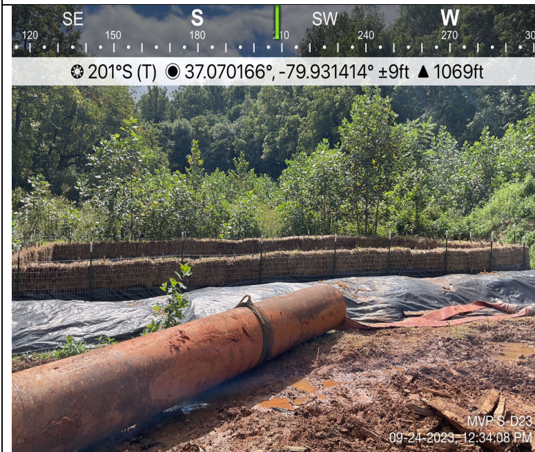
Photo Description: Dewatering structure set up in upland area and discharging onto vegetated area.
