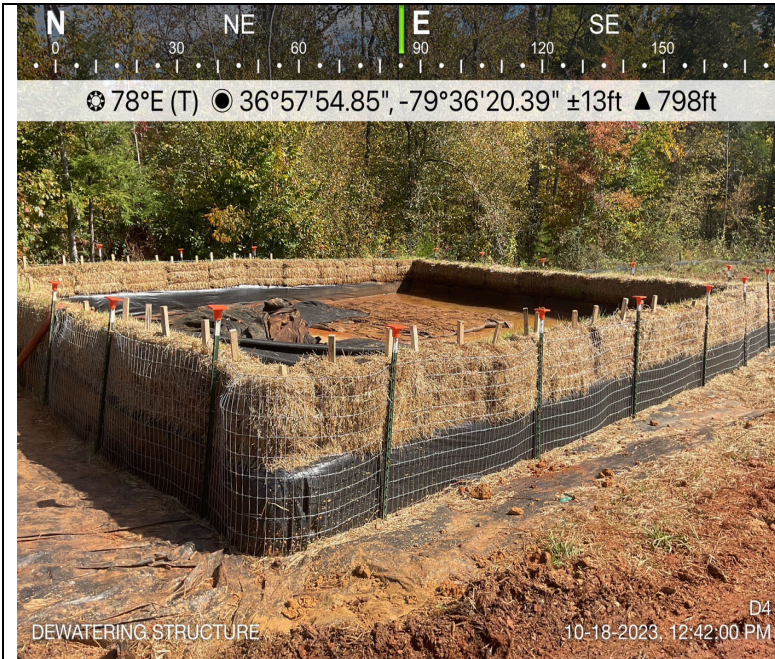
Photo Description: Overview of the Dewatering structure.
