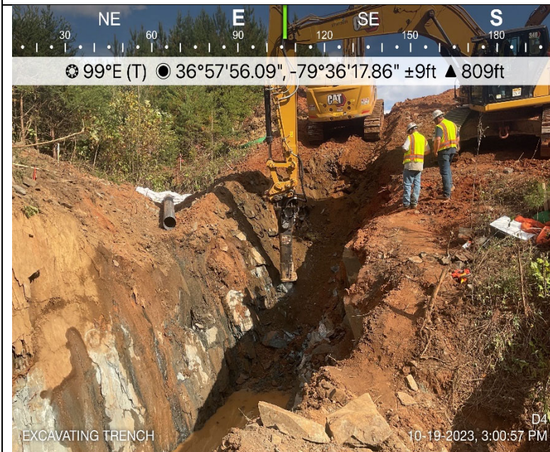
Photo Description: Excavation of the trench.
