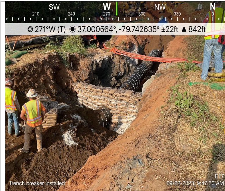
Photo Description: Trench breaker installation.
