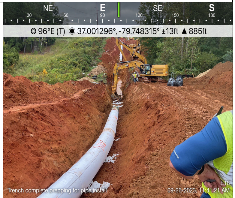
Photo Description: Trench open and pipe laid across the resource.
